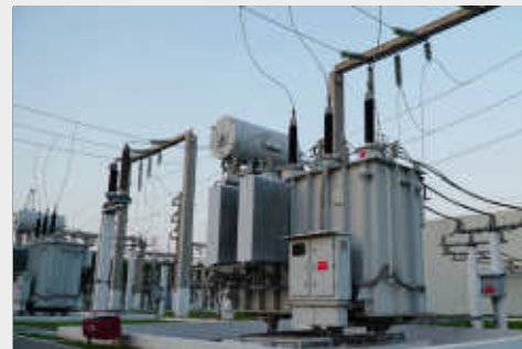
33/11kV Substation featuring 2x8 MVA transformers with TPCODL in Odisha
