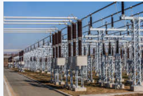
Data Centre substation & line - construction of 220/33 KV GIS Substation and associated Transmission line
