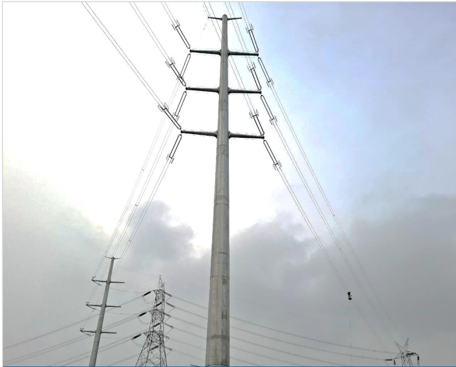
Jalpura – Khurja 400kV D/C transmission line
