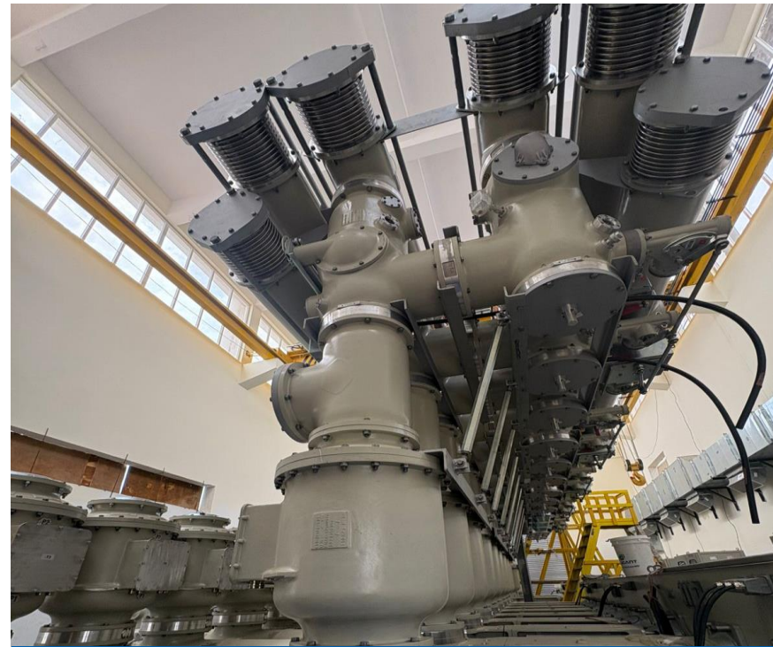
400/220 kV GIS substation at Metro Depot & Jalpura
